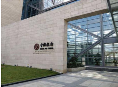
BMS of China Bank
