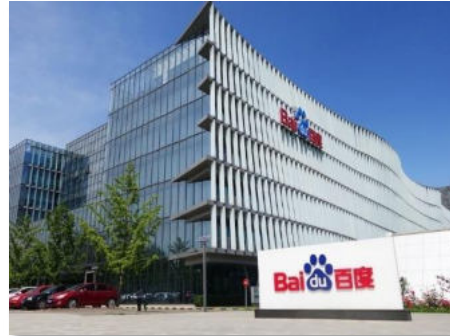
BMS of China Baidu Data Center
