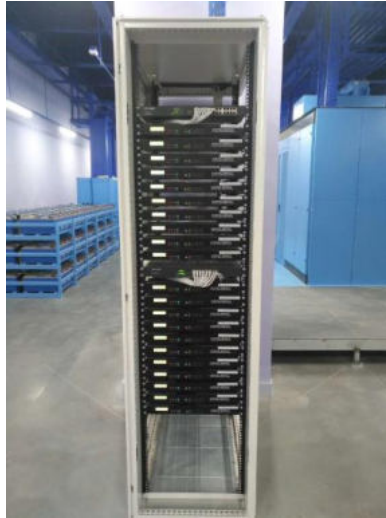
Control module installation
