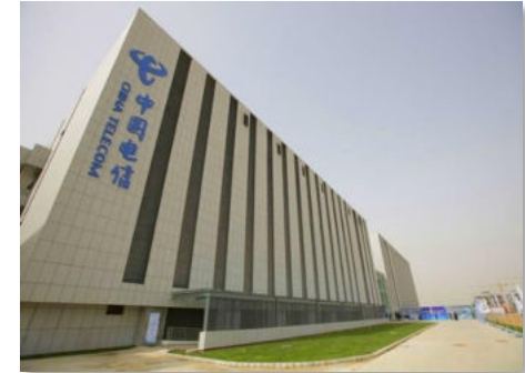
BMS of China Baidu Data Center
