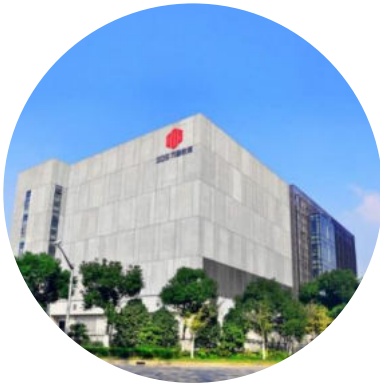
BMS of Data Center
