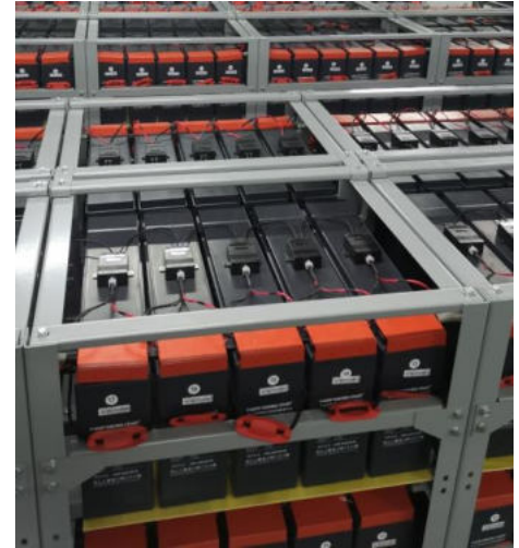
Sensor installation
